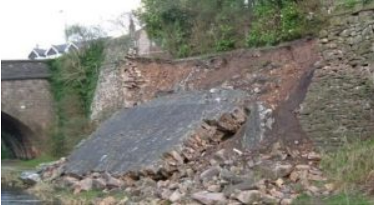
Figure 7.13. A failed retaining wall. Ray Folwell, CC BY-SA..
