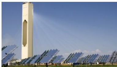
Figure 10.31. Thermal solar power generation with a solar power tower. Afloresm, CC BY.
