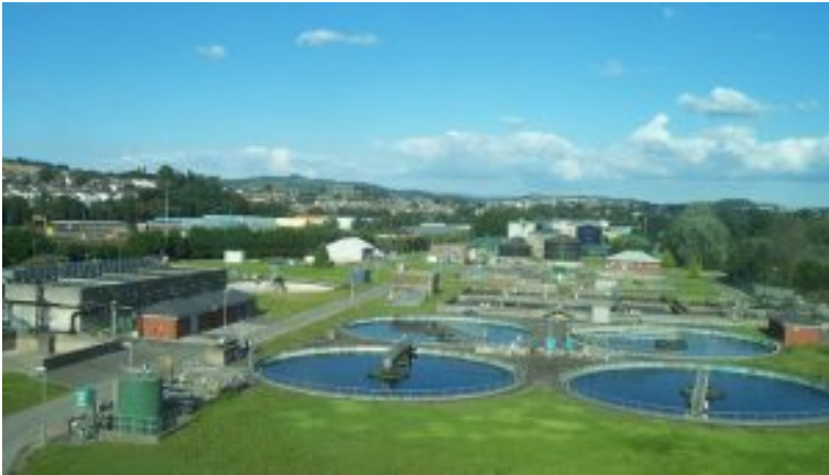
Figure 11.15. Photo of a typical municipal sewage treatment facility. Each of those settling tanks is approximately 15 meters in diameter and 3 meters deep. Everything is connected via underground pipes. Lewis Clarke, CC BY.
