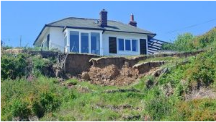
Figure 7.10. Construction and erosion have combined to steepen this slope, making it increasingly unstable with time. Obviously, the house is in serious trouble. Wilson44691, Public Domain.
