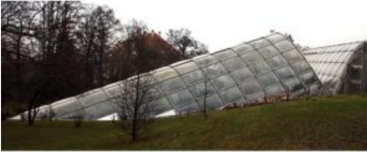
Figure 10.29. Passive solar heating. Use of sun-facing glass maximizes energy absorption and heating of this building. Marion Schneider & Christoph Aistleitner, Public Domain.
